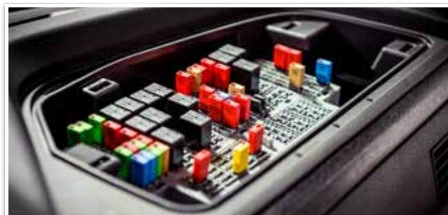
In-cab electrical panel
